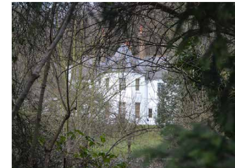
Fig. 20: Large Residence - Old Vicarage
