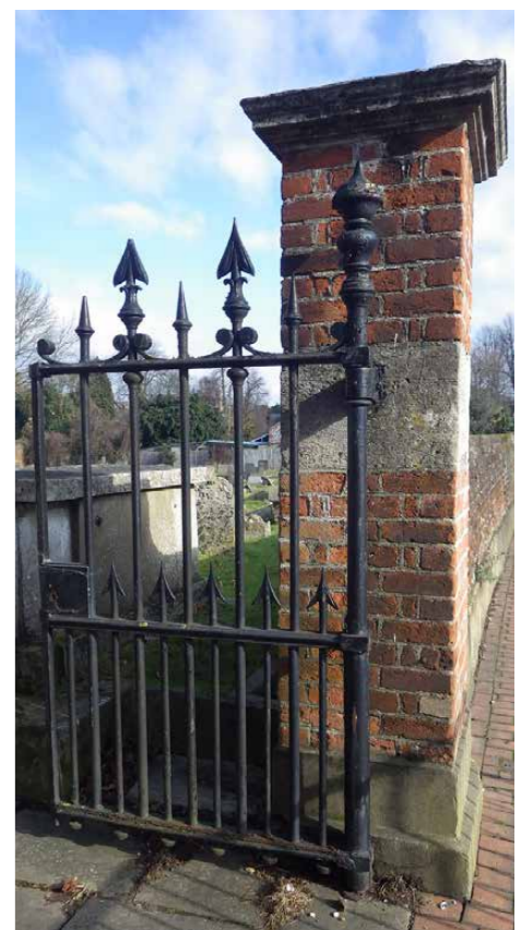
Figure 29: Gate and brick wall to churchyard.
